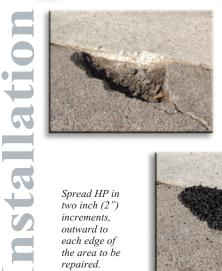
Clear pothole of loose debris and pour HP into the hole or utility cut.
